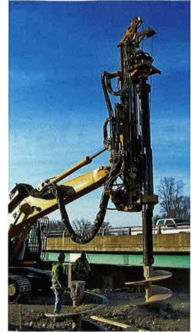
Photo: GeoDrill 7000 at the construction site at Gurnee, Illinois
